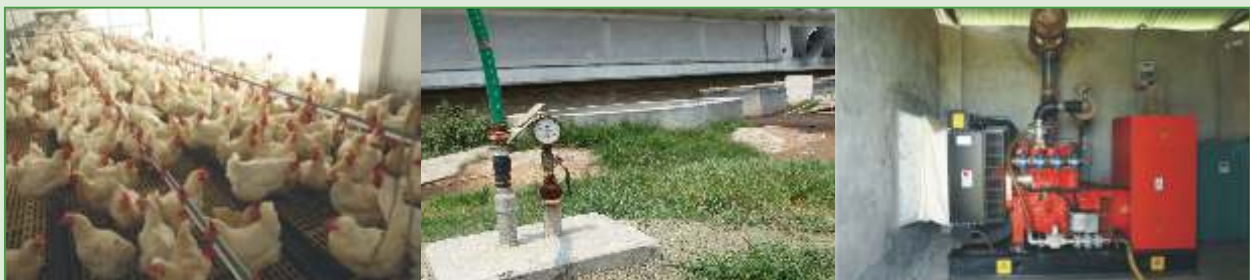
Large farms can produce electricity with captive biogas-powered generators. The produced biogas, can be also used as a clean fuel for cooking and lighting
