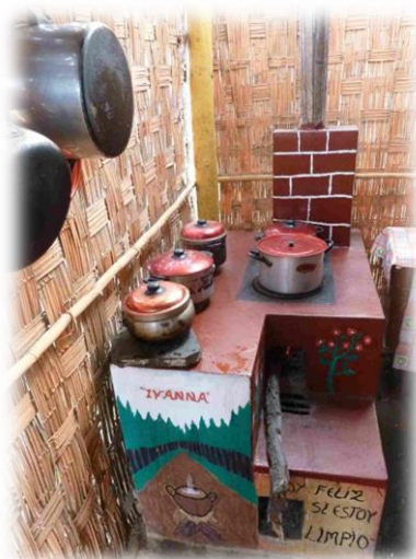
Typical improved in situ construction stove. The stove has been decorated by the family post project.
