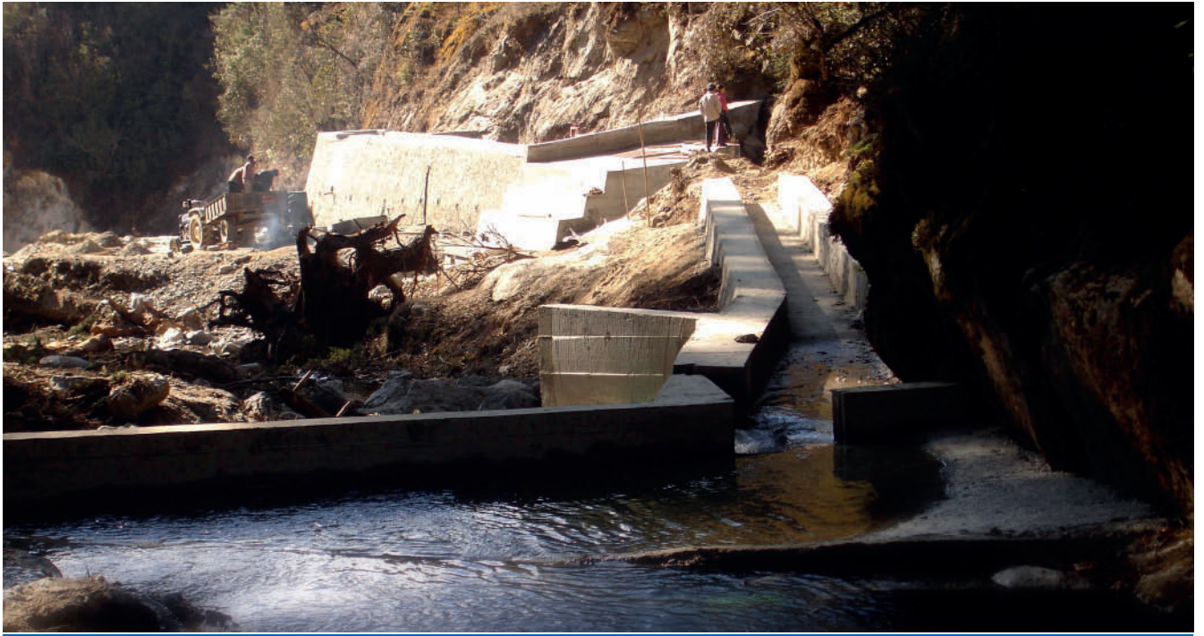
A view of the intake diversion canal. Project: Community Micro-hydro for Sustainable Livelihoods – Sengor, Bhutan.
