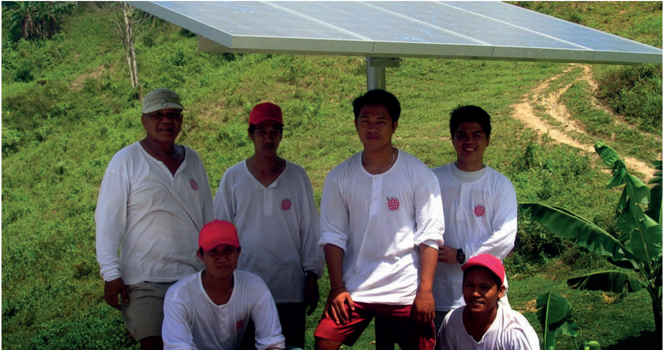
Erecting a solar photovoltaic system. Project: Accelerating Community Electricity Services using Solar (ACCESS) – the Philippines.
