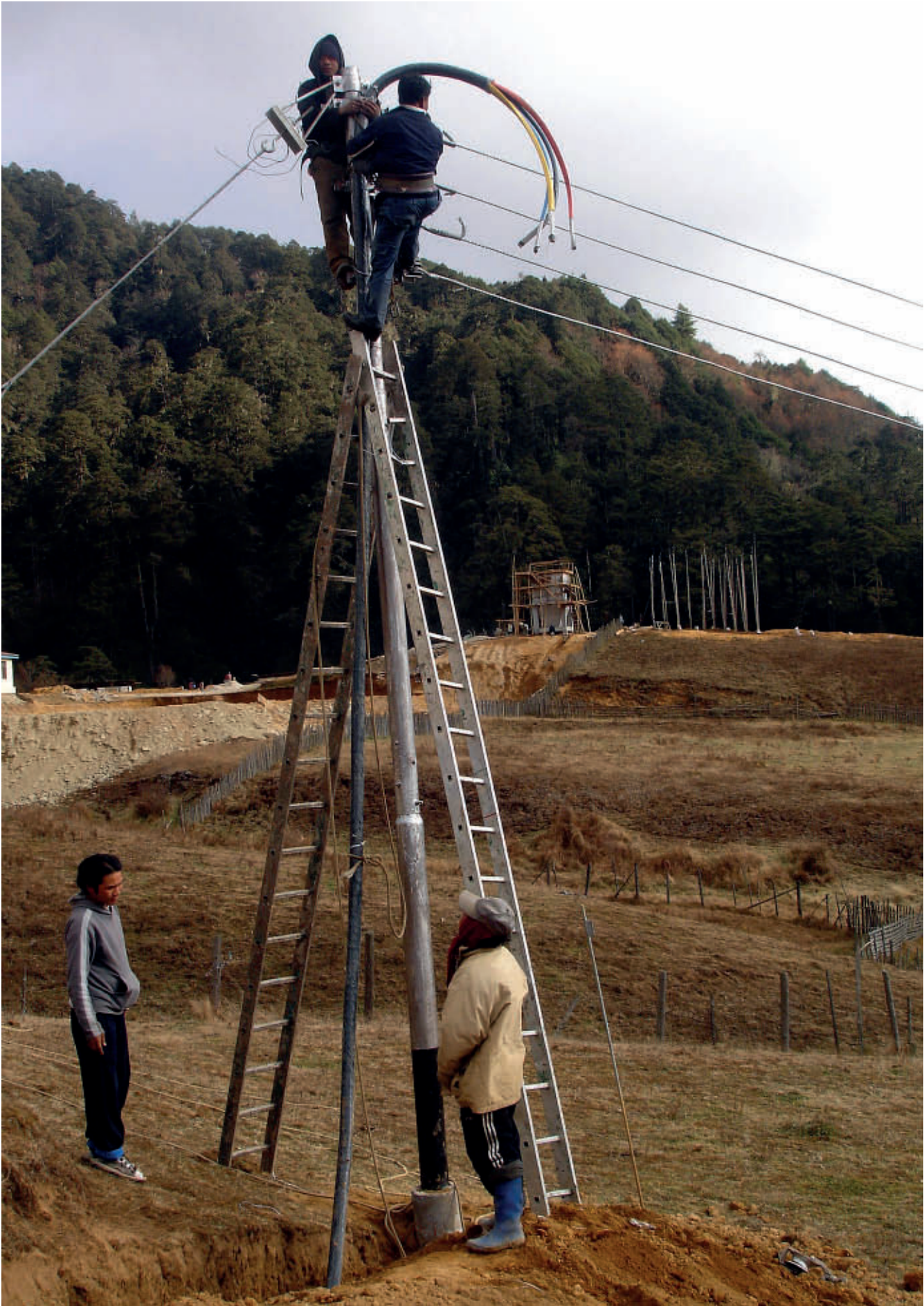
Wiring for household electrification. Project: Sengor – Bhutan.
