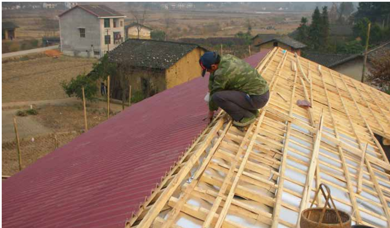
A double layer aluminum roof improves the “thermal envelope” of a house in Hunan Province, China helps to reduce heating requirements. (Credit: He Jianqing)
