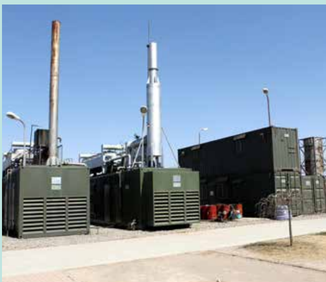
A power generator that uses captured landfill gas in China. (Credit: Yang Aijun/WorldBank)
