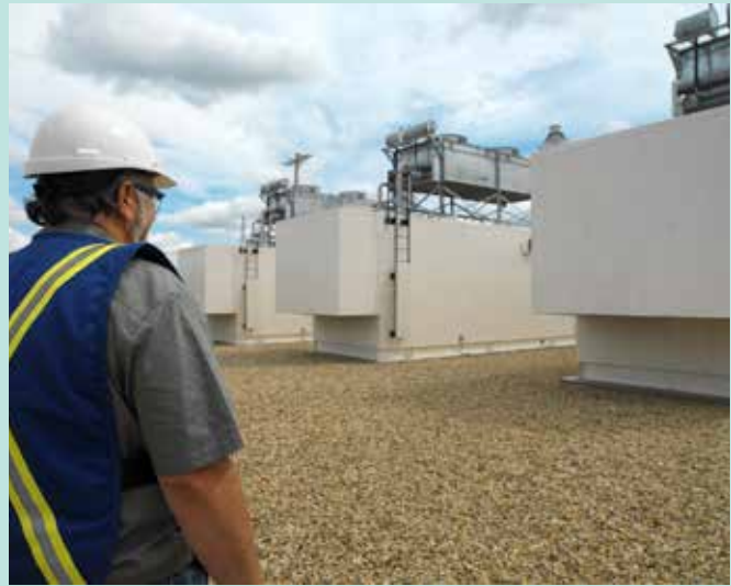
Electricity generators use landfill gas as fuel in Edmonton, Canada. (Credit: Pembina Institute)
