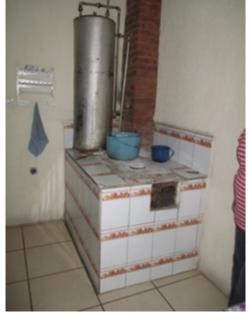
Plancha stove with water heater attached (replaced LPG stove)
