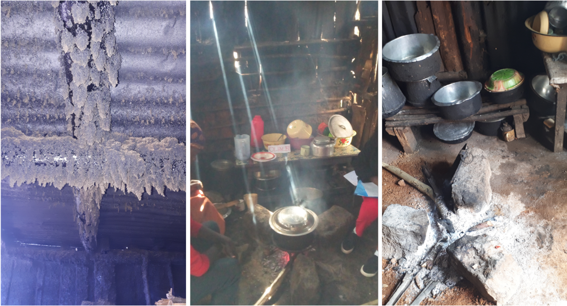
Figure 19: (Left to right) 1) smoke damage on the ceiling of a participant's cooking area, 2) smoke levels in a participant's cooking area, 3) storage of kitchen utensils
