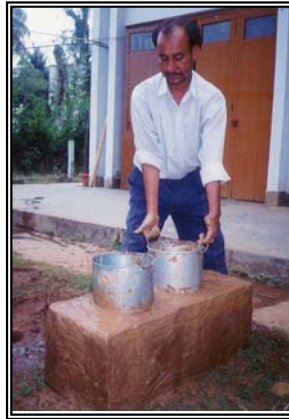
Figure No: 13 2 nd Stage: Construction of Double Mouth Cooking Stove (on the floor)
