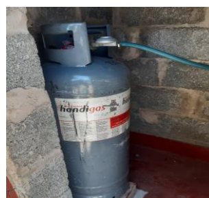
Figure 12 LPG cylinder secured in a concrete block housing at a respondent's house
